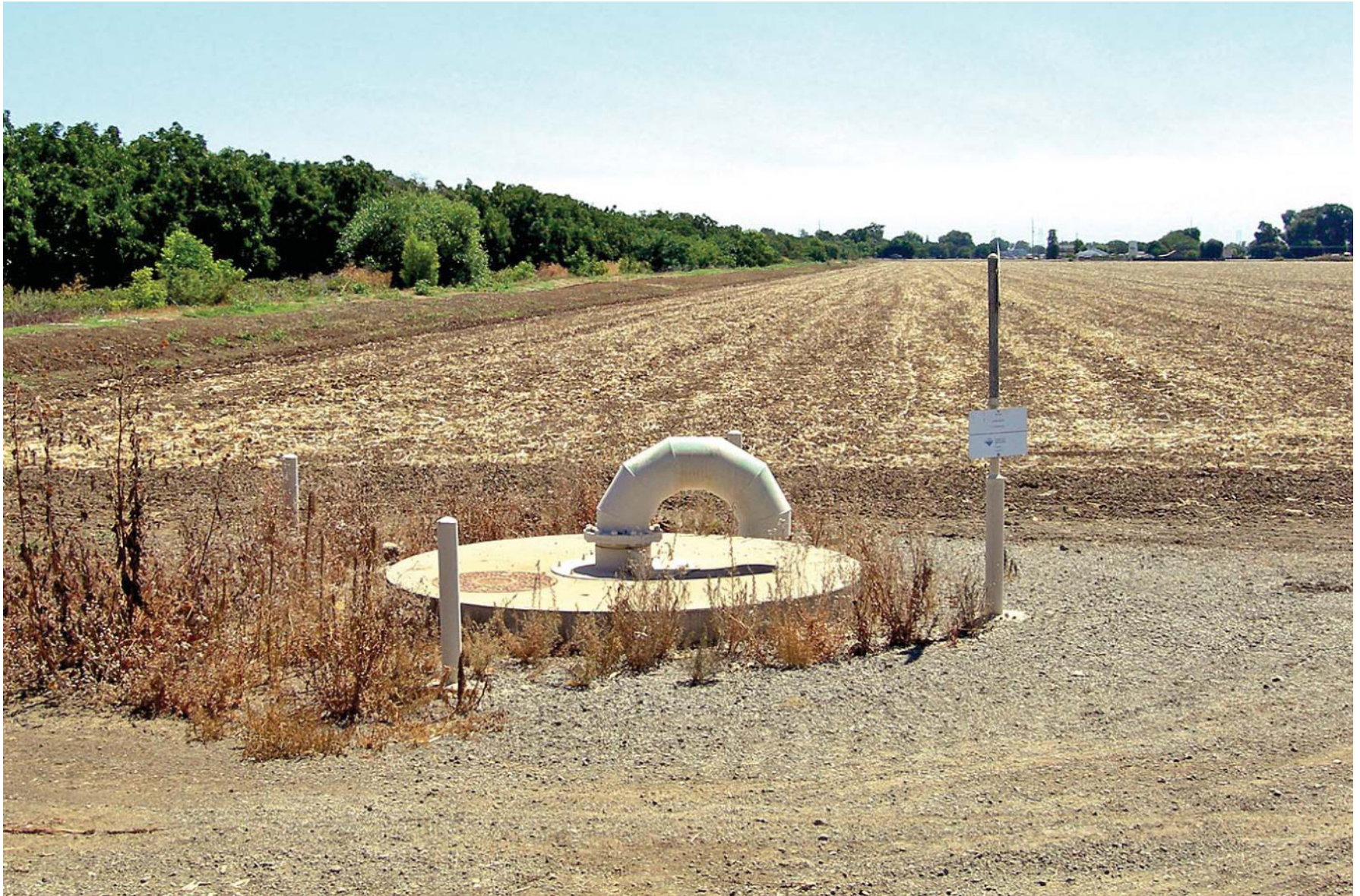
Figure 3-9 Example of Typical Air Relief Valve Structure
